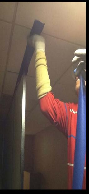
Set ceiling channel then drop line to set floor angle
